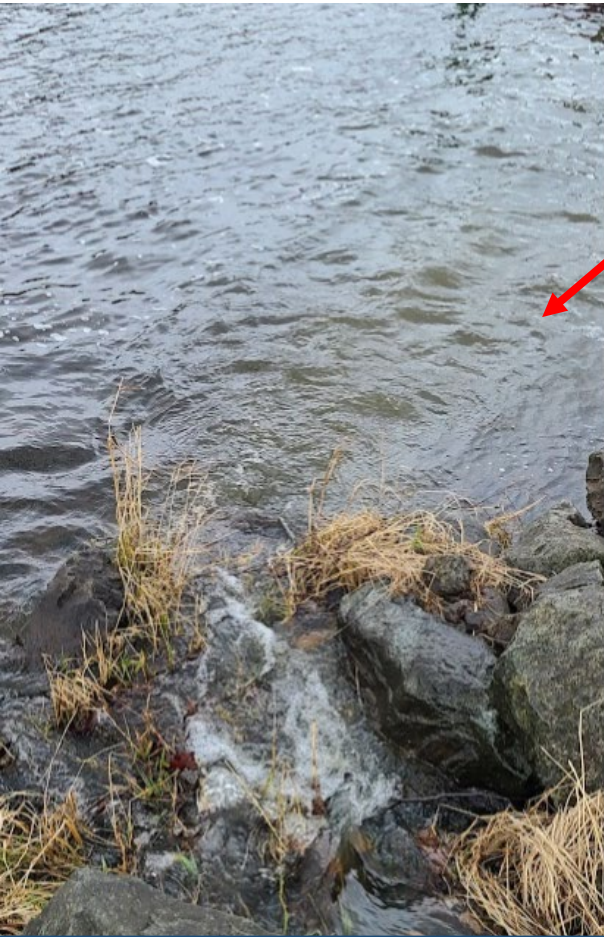
Big Lake Outfall receiving sediment-laden water from Overlook Crest
